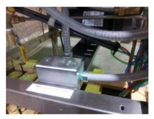
AFB connection box, the water inlet can be seen at left
