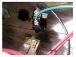
Optional Chemical Alarm switch, buzzer
